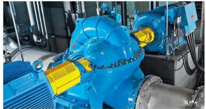
ANDRITZ double-suction axial split case pump operating as headbox pump © ANDRITZ
