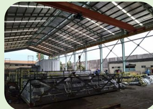
Fabrication Area (Crane Up To 20 Tons)
