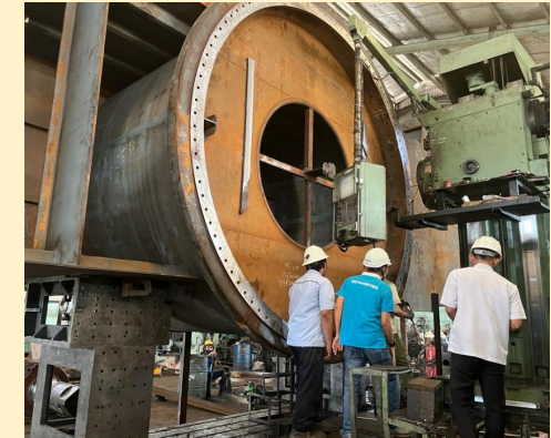
Beam Crane Milling dimension 8000mm
