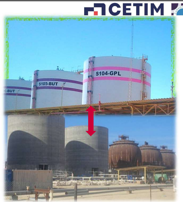
Gas storage spheres under sarcophagus (with wave guides)
