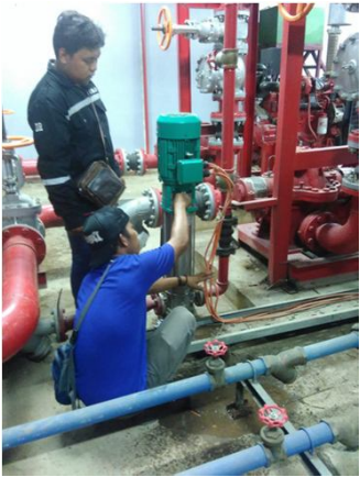
Pemasangan Pompa Hydrant & Jockey Pump
