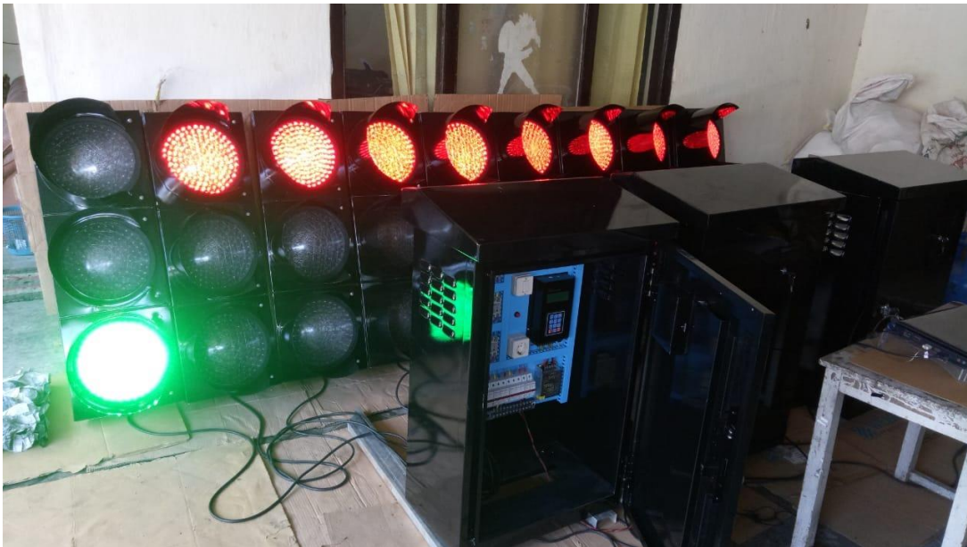
INSTAL LAMPU TRAFFIC LIGHT
