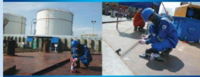
MAGNETIC PARTICLE INSPECTION TESTING
