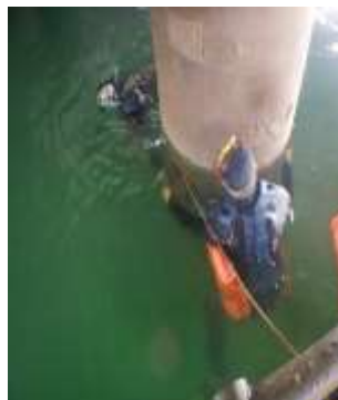
Apr 2021 - Jacketing for Jetty Pile - TBBM Bau Bau, Sultra
