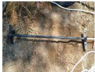
Instalasi Anode Centralizer
