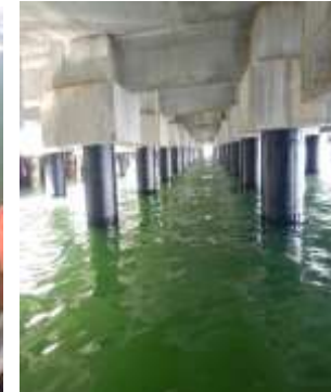
Apr 2021 - Jacketing for Jetty Pile - TBBM Bau Bau, Sultra
