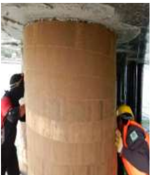
Apr 2021 - Jacketing for Jetty Pile - TBBM Bau Bau, Sultra
