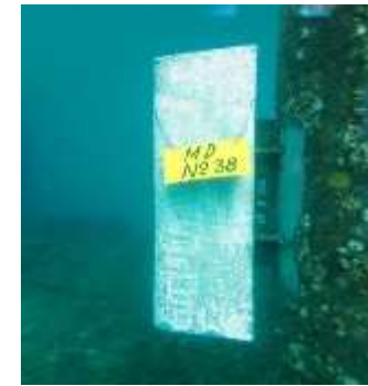
Mar 2021 - Sacrificial Aluminium Anode for Jetty Pile - PLTU Bolok, Kupang, NTT
