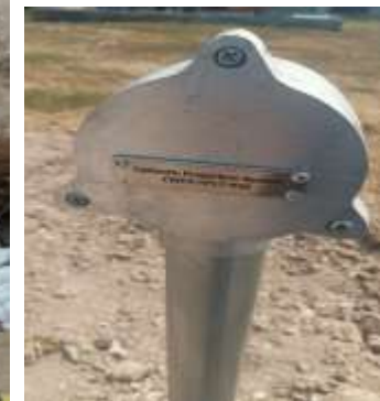
2018 - Sacrificial Magnesium Anode for Underground Pipeline - PLTU Sebalang 2 x 100 MW, Lampung
