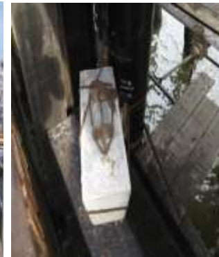
May 2015 - Sacrificial Aluminium Anode For Jetty Pile - PT Chevron Indonesia, Dumai, Riau
