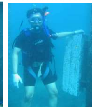
2008 - Sacrificial Aluminium Anode for Jetty Pile - PLTU Jawa Tengah 2 x (300-400 MW), Rembang, Jateng
