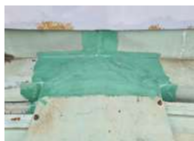
Maret 2022 - Perbaikan Atap Gudang with Water Shield, Reinforced Fiber Glass - PT. Lotte Chemical Titan Nusantara
