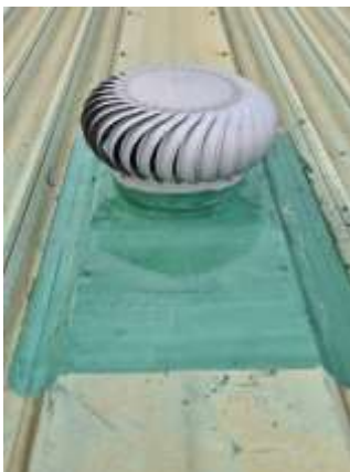
Maret 2022 - Perbaikan Atap Gudang with Water Shield, Reinforced Fiber Glass - PT. Lotte Chemical Titan Nusantara
