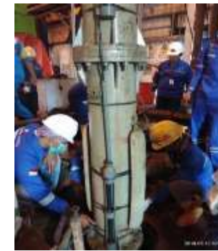
2018 - Sacrificial Aluminium Anode for Cooling Water Pump - PLTU Indramayu 3 x 350 MW, Indramayu, Jawa Barat
