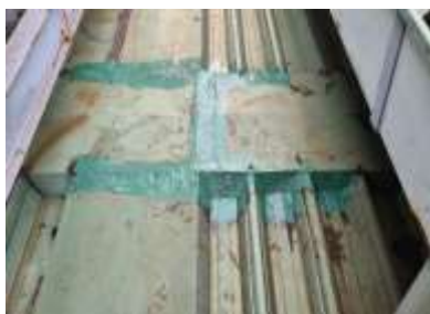
Maret 2022 - Perbaikan Atap Gudang with Water Shield, Reinforced Fiber Glass - PT. Lotte Chemical Titan Nusantara
