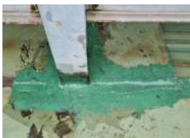
Maret 2022 - Perbaikan Atap Gudang with Water Shield, Reinforced Fiber Glass - PT. Lotte Chemical Titan Nusantara
