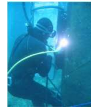
2008 - Sacrificial Aluminium Anode for Jetty Pile - PLTU Jawa Tengah 2 x (300-400 MW), Rembang, Jateng
