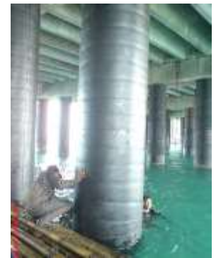
2012 - Jacketing for Jetty Pile - PT. Indonesia Power, Suralaya, Merak, Banten
