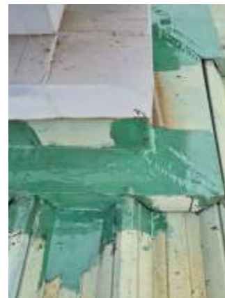
Maret 2022 - Perbaikan Atap Gudang with Water Shield, Reinforced Fiber Glass - PT. Lotte Chemical Titan Nusantara
