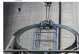
KILN SHELL REPLACEMENT (PT SEMEN BATURAJA), 2014
