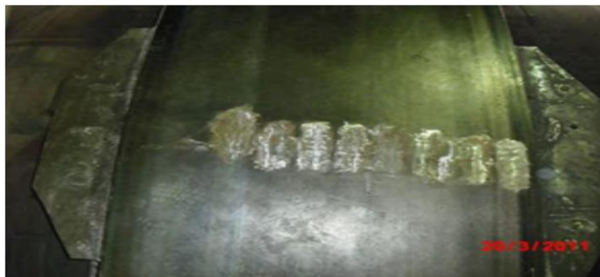
CRACK REPAIR ON KILN TIRE (PT. SEMEN INDONESIA, TUBAN) 2011
