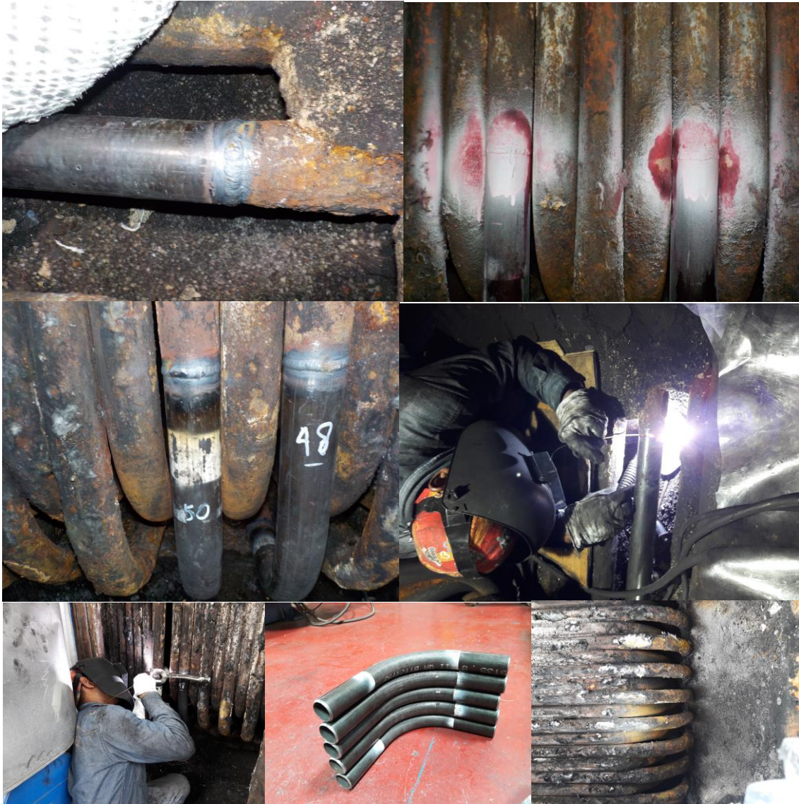
RETUBING PARTIAL START UP BOILER – PLTU INDRAMAYU - 2016
