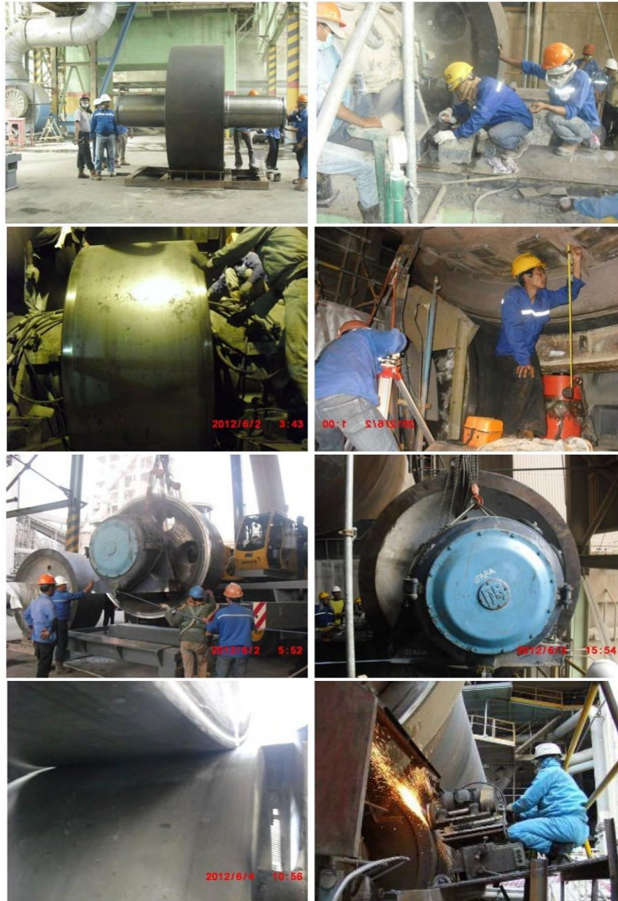
SUPPORTING ROLLER REPLACEMENT (PT. SEMEN INDONESIA TUBAN I), 2012
