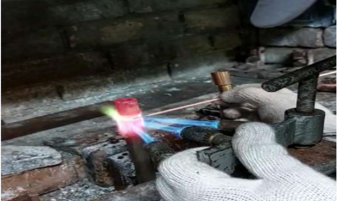
Pipe Copper / Brazing
