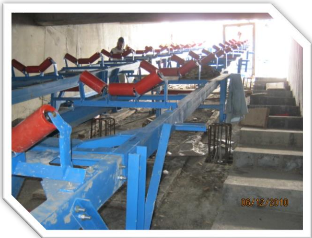
INSTALL ROLLER CONVEYOR
