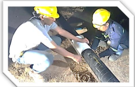
WRAPPING UNDERGROUND PIPE
