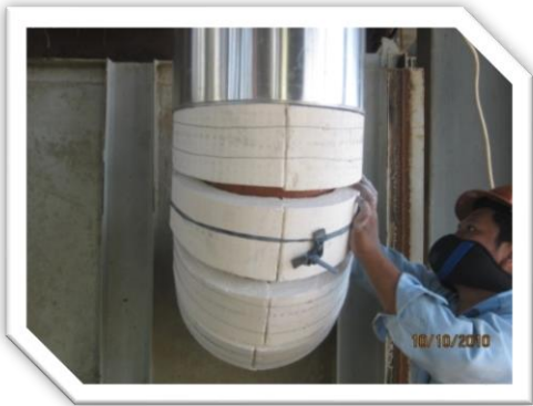
INSULATION ELBOW
