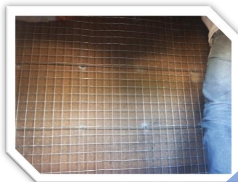
INSTALL WIRE MESH
