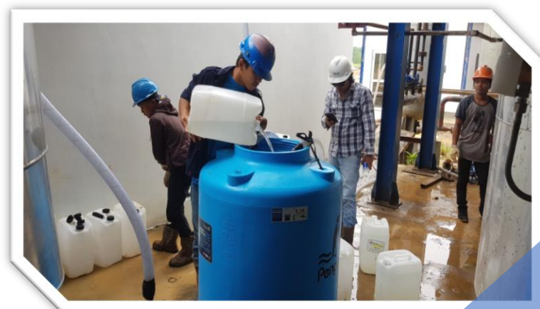
INJECT CHEMICAL FOR CLEANING BOILER
