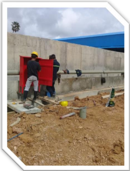
INSTALL HYDRANT BOX
