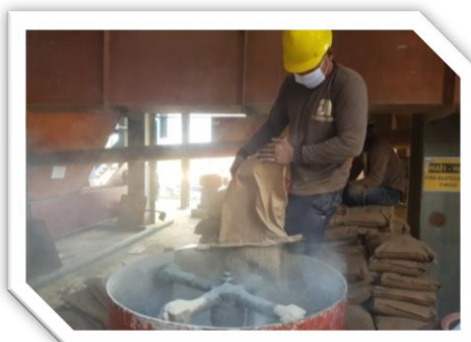
MIXING PROCESS OF CASTABLE MATERIAL
