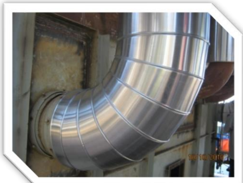
INSULATION ELBOW
