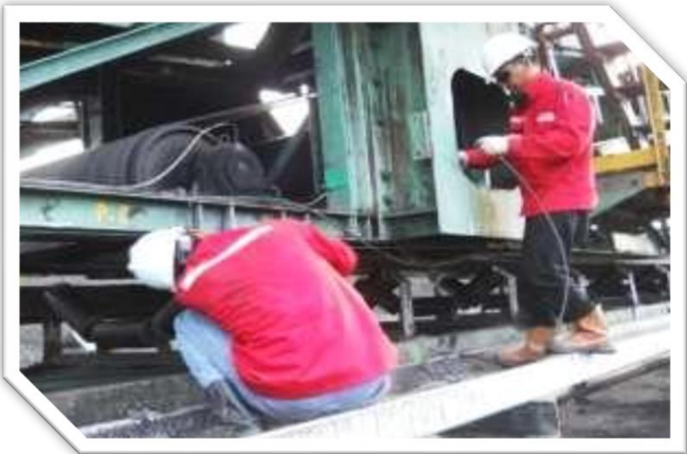
INSTALL BELT CONVEYOR
