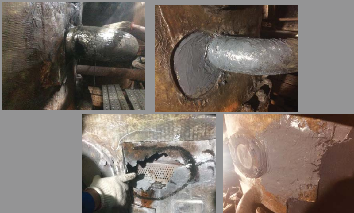
REPAIR CONDENSOR PIPE LEAKAGE AT PT. INDONESIA POWER PNS
