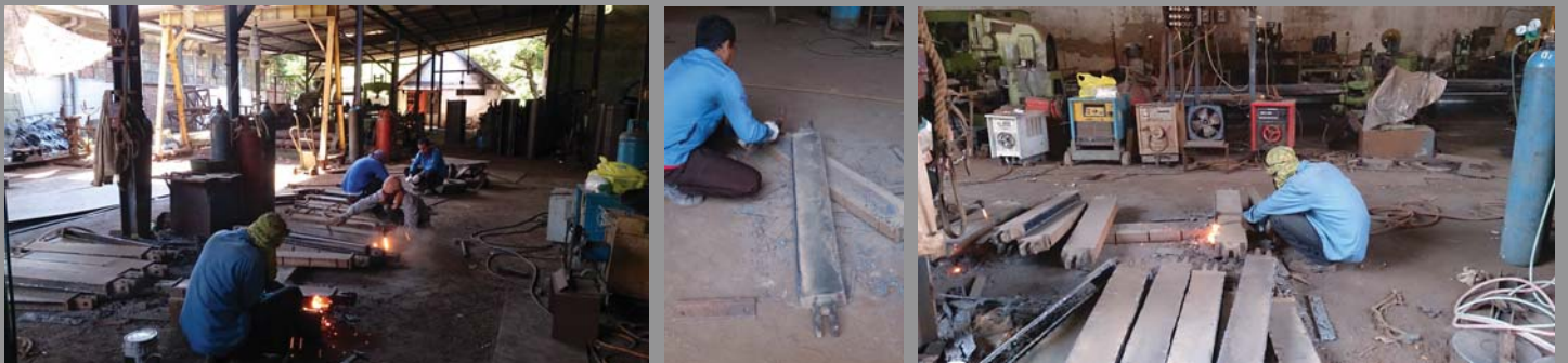
REPAIR CONDENSOR PIPE LEAKAGE AT PT. INDONESIA POWER PNS
