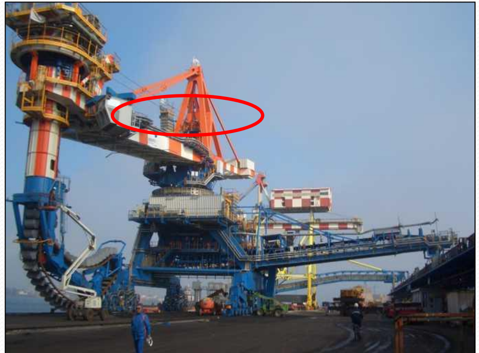
Rotational chain system (in the red circle)
