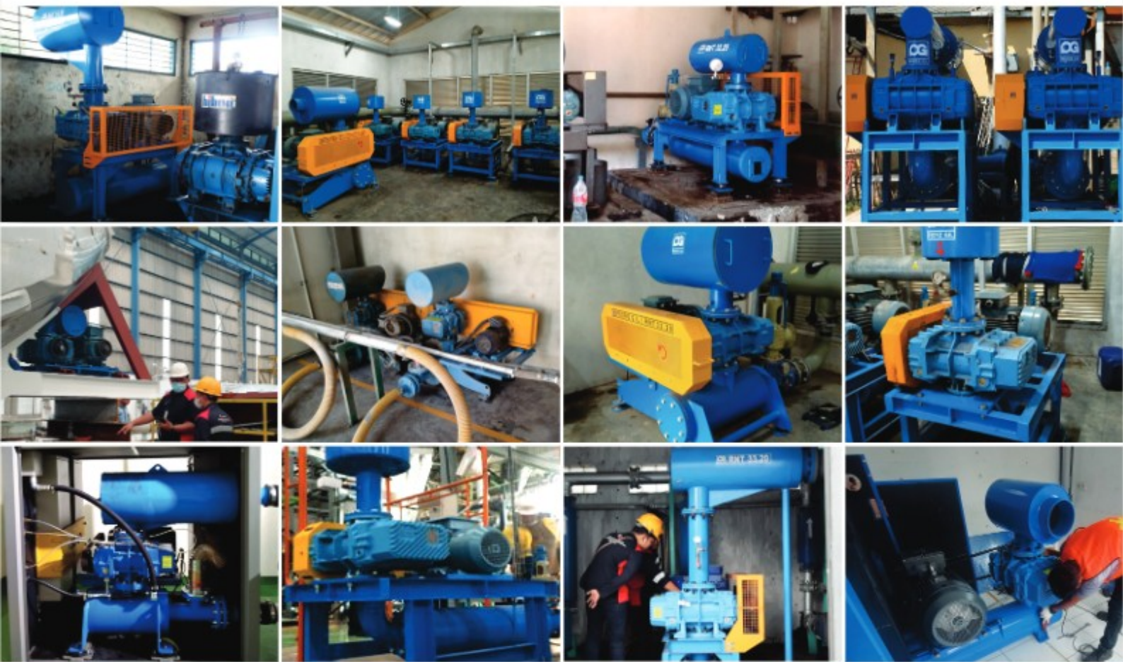
New Installation Of Pedro Gil
