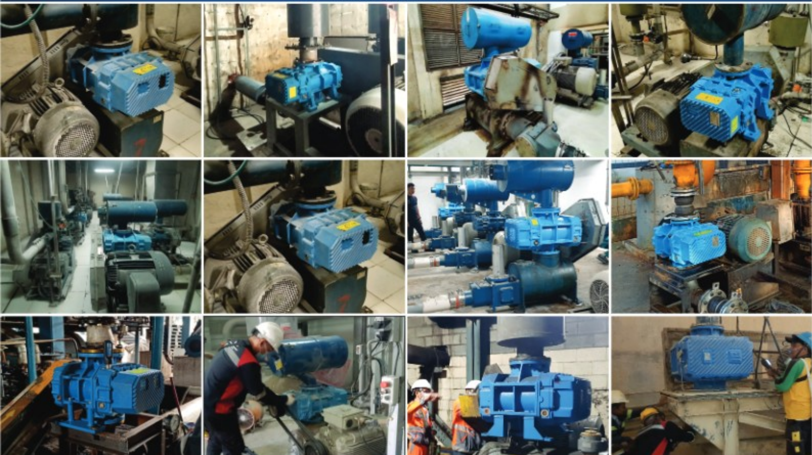
Pedro Gil Installed at Existing Baseplate
