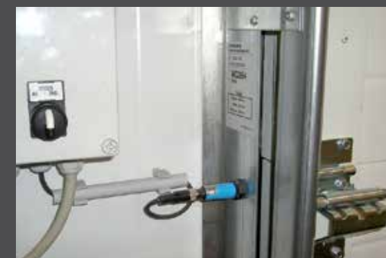
SENSORE PER INTERCONNESSIONE RAMPA-PORTONE DOCKLEVELLER-DOOR CONNECTING SENSOR
