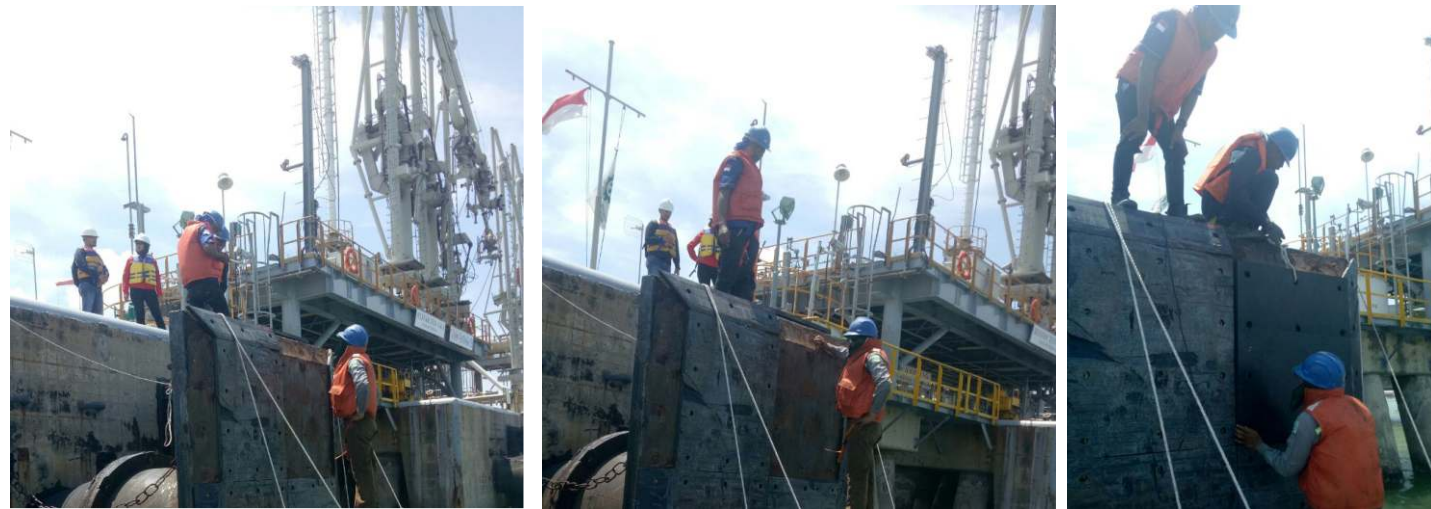
Repair Chain and Pe Pad
