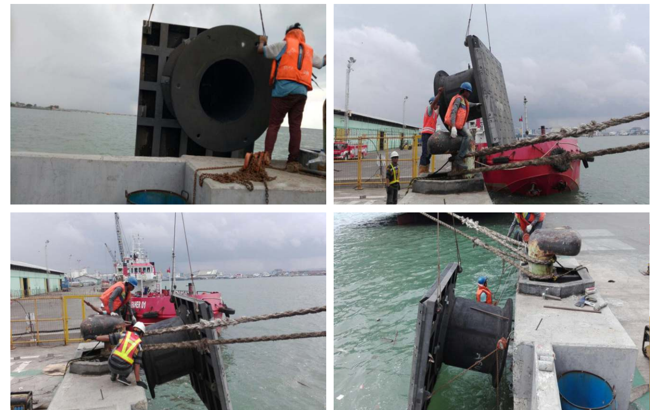
Frontal Frame Installation
