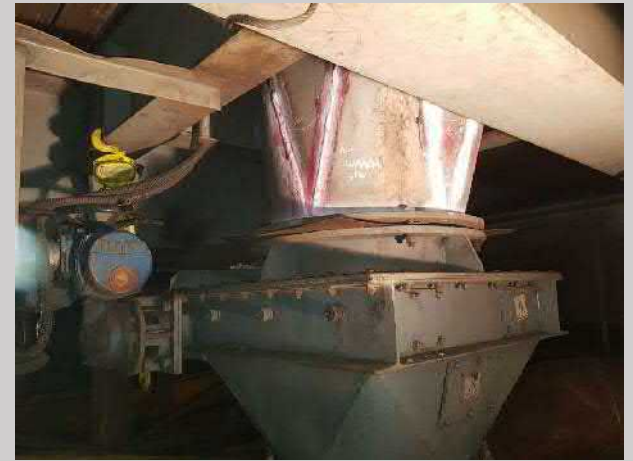
NDT Check & Finishing
