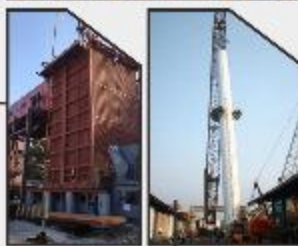
INSTALASI BOILER CHAINGRATE 30 TON 2 UNIT
