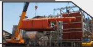
ERECTION & INSTALLATION BOILER 30 TON
