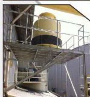
FABRICATION PLATFORM COOLING TOWER
