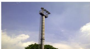
Tower Pabrik PT. Bir Bintang, Mojosari Pasang Tunnel
