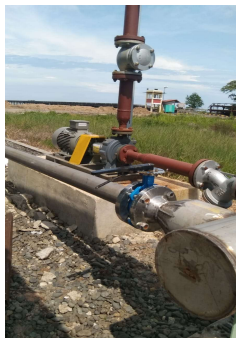
WWTP Pump with VFD 7.5kW – ABB
