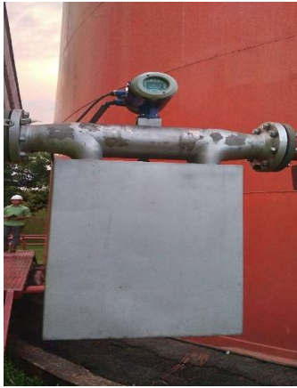
Replace Coriolis Mass Flow meter 4in – 250 m 3 /h
