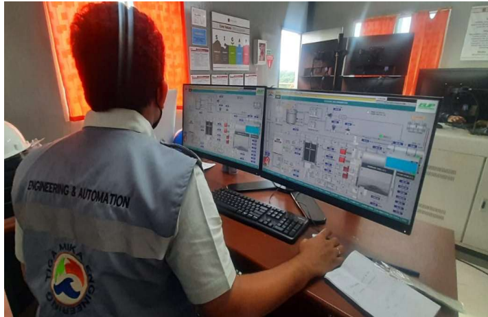
Thermax Boiler NEW SCADA – HMI PC- SIEMENS
