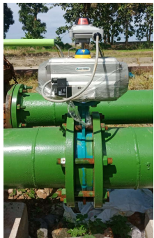
Pneumatic Actuator Butterfly Valves 8in
