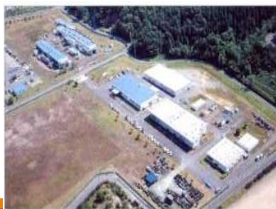
Shiga Plant Established October, 1986. Produces undertakes resin processing of core cord for power transmission belts.
