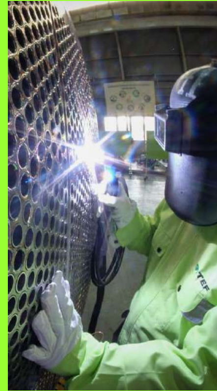
匠の溶接 Workmanship (Proficiency in Welding)
