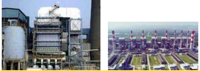
FGD system for Power Plant
