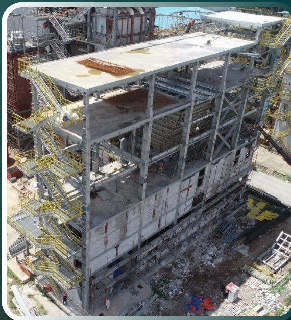
STEEL STRUCTURE FOR BOILER
