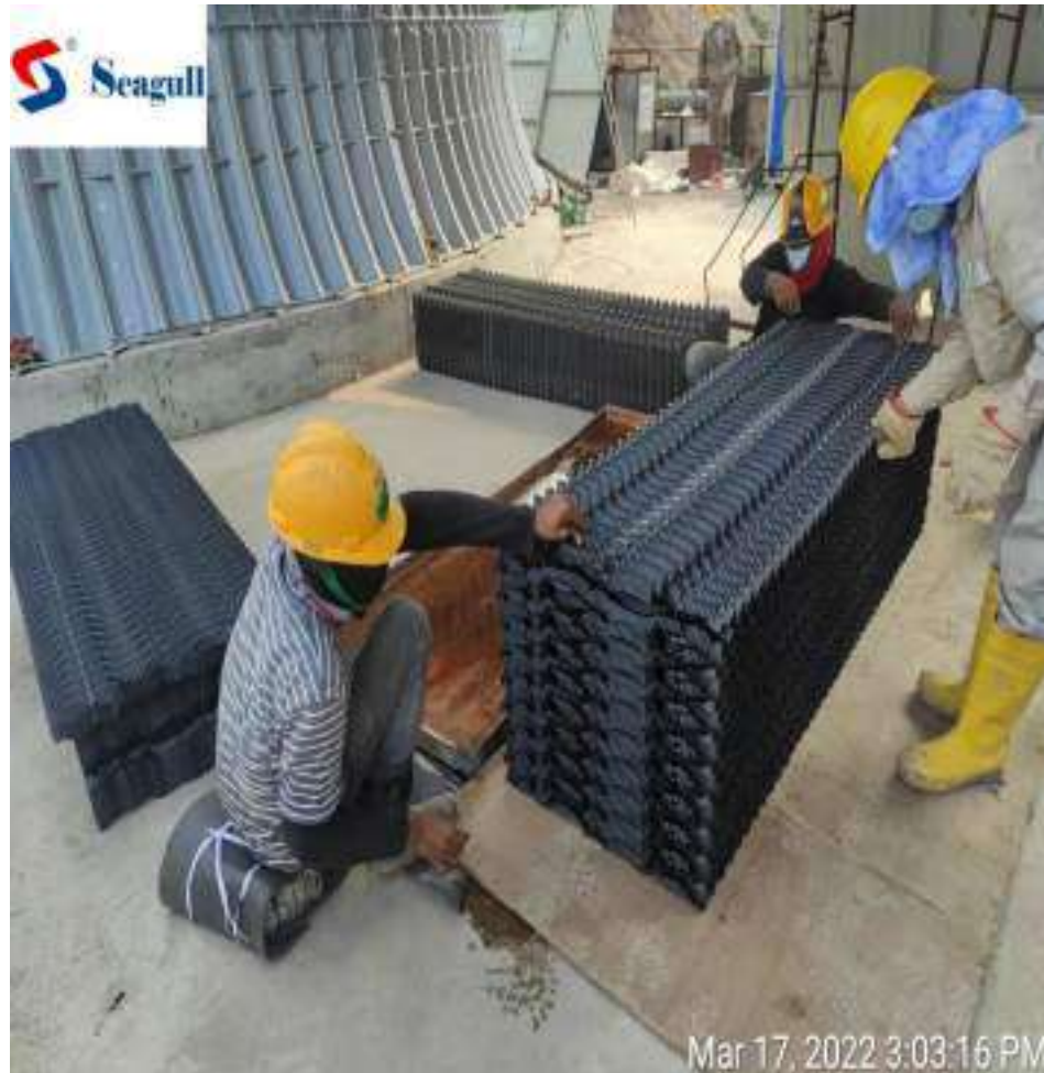
Infill Bonding
