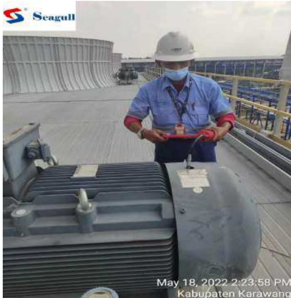
Re-greasing Motor Before Commissioning
