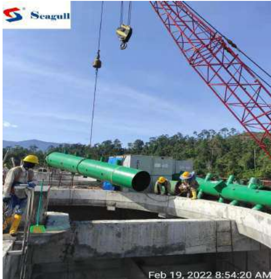
Header pipe installation
